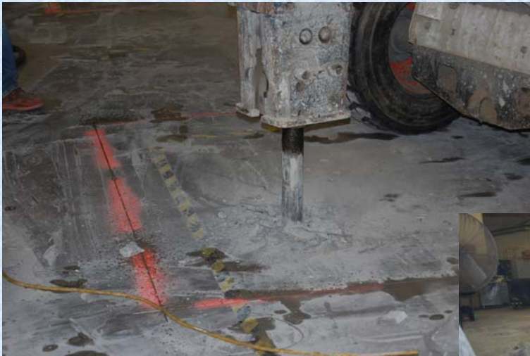
MGI breaks ground for the new manufacturing system.
